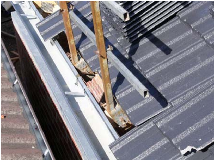
Figure 9.8.6 – Method of attachment of perimeter fencing
