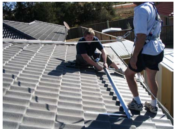
Figure 9.8.3 – Roofers with safety harness and lanyard
