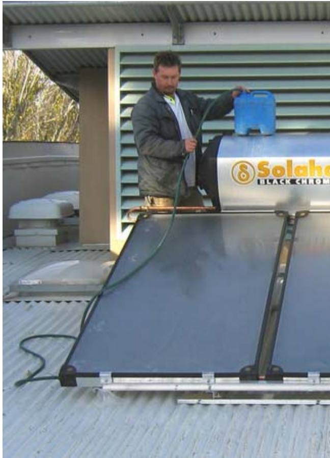
Figure 9.11.1 – Charging the collectors and jacketed tank with anti-freeze solution
